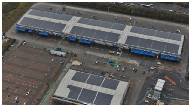
Figure 9: Ariel view of solar PV array installed on the Western International Market supported by Hounslow Council.
