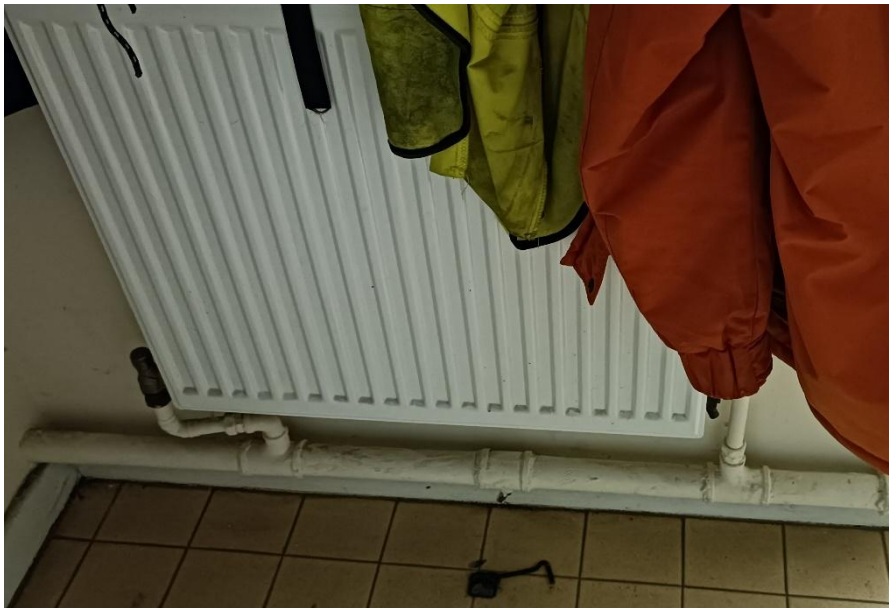
Figure 15 Single-pipe Heating System: Anytown Crematorium
