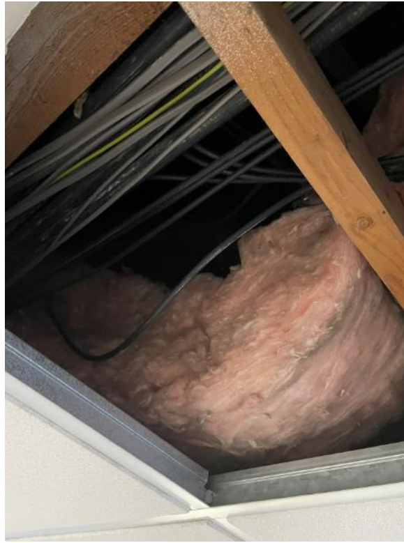
Figure 18: Existing Loft Insulation (~150mm)
