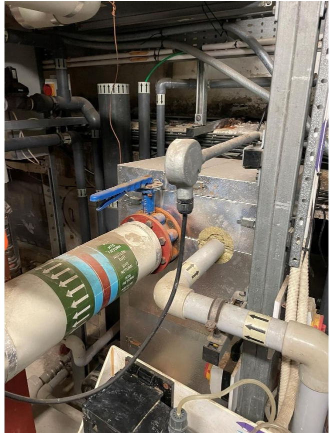
Figure 23: Learner Pool Plate Heat Exchanger (Left) & Main Pool Plate Heat Exchanger (Right)
