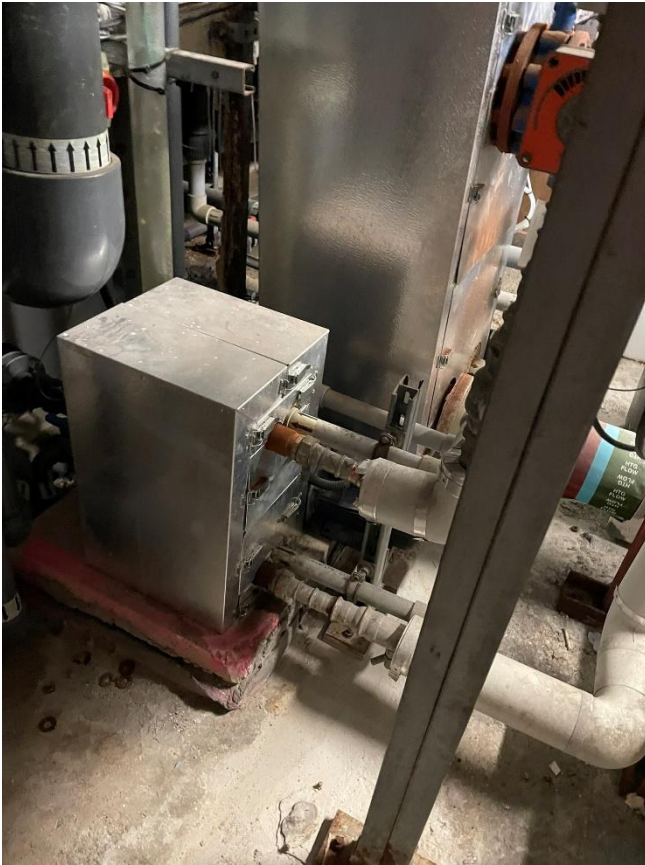
Figure 23: Learner Pool Plate Heat Exchanger (Left) & Main Pool Plate Heat Exchanger (Right)
