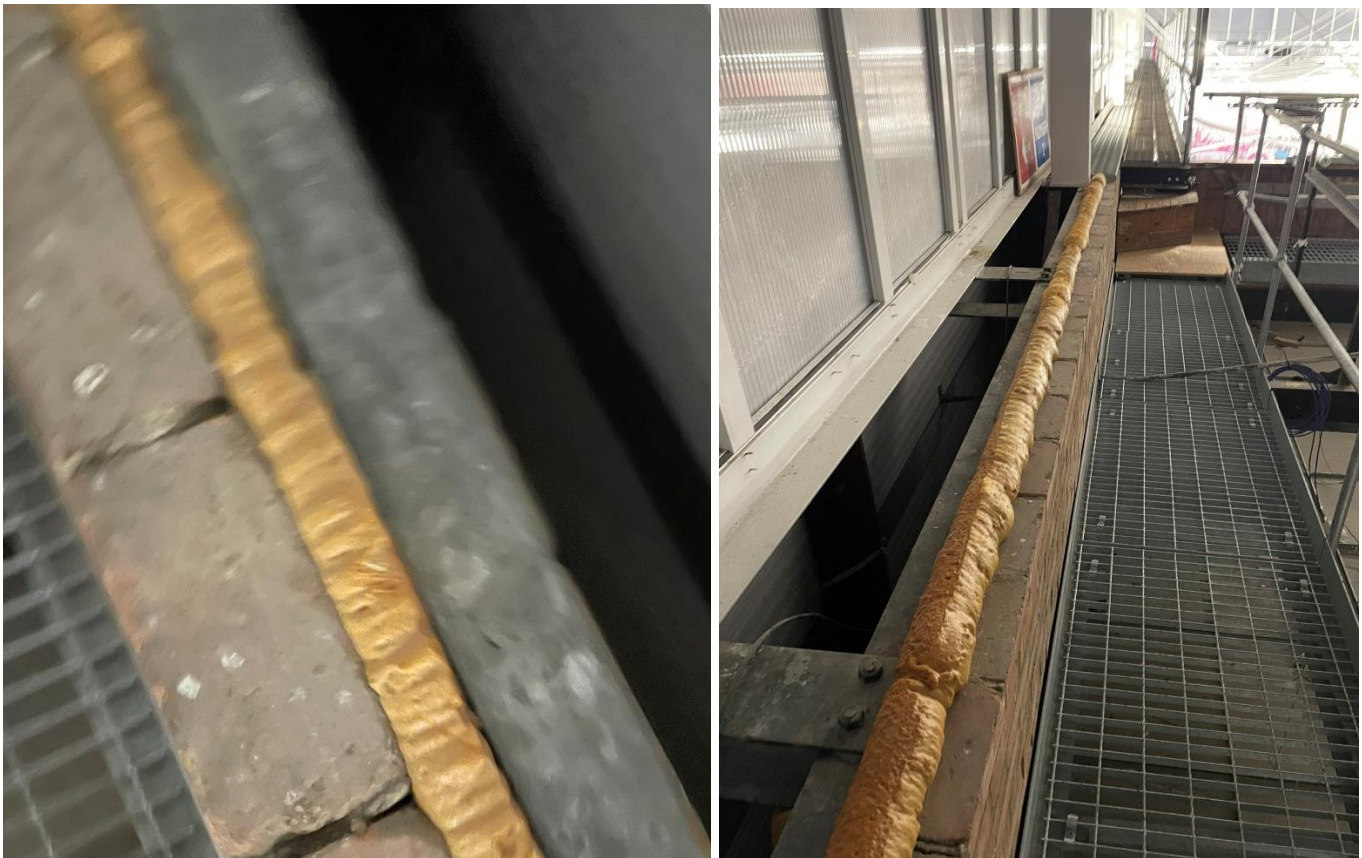
Figure 51: Ice Rink Wall Construction
