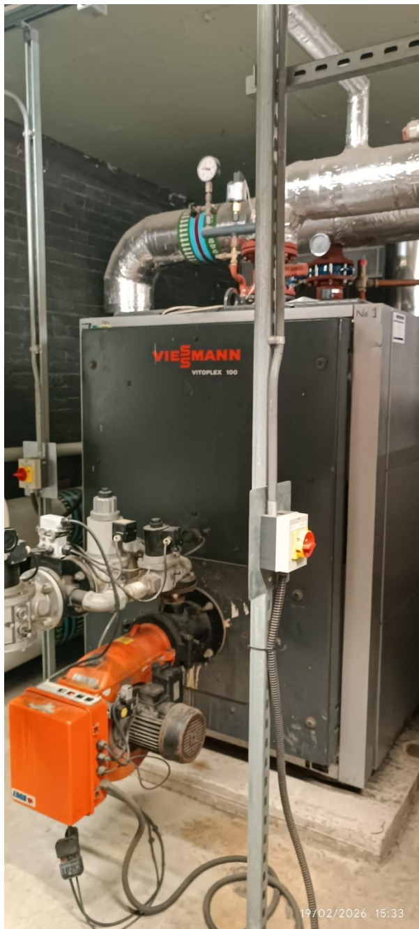
Figure 24: 2no. Viessmann gas boilers (2004)
