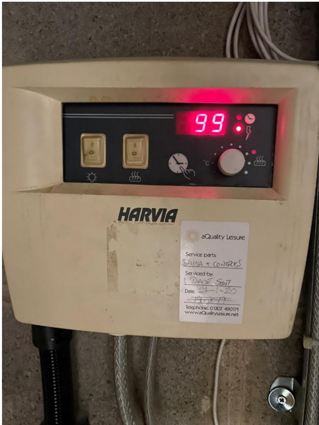
Figure 41: Harvia Sauna Controller
