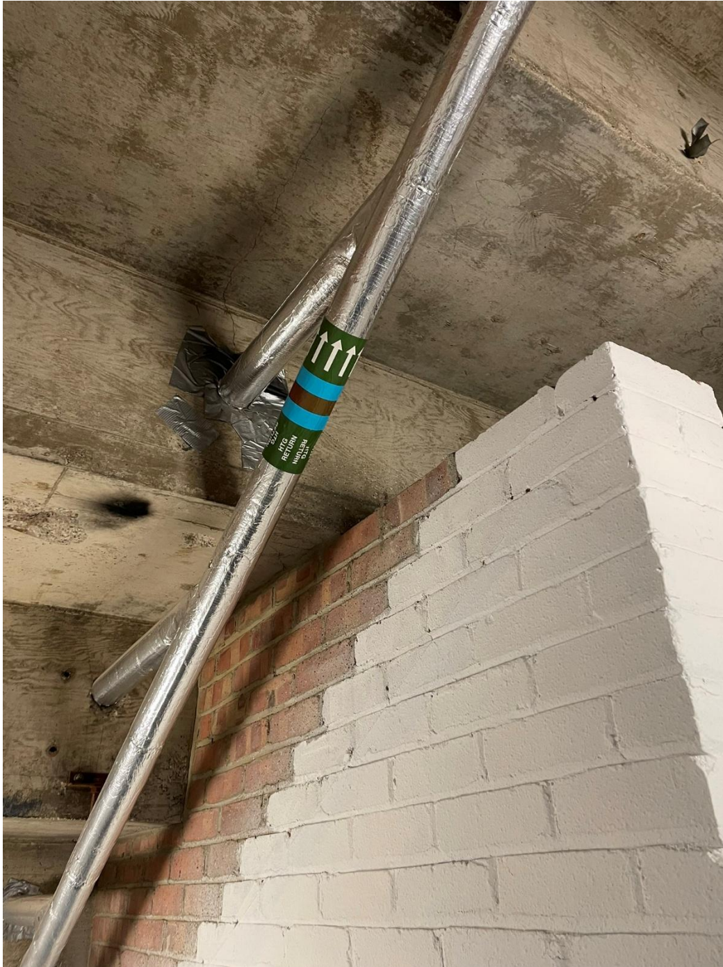
Figure 35: Heating circuit under Ice Skate Spectator Seating
