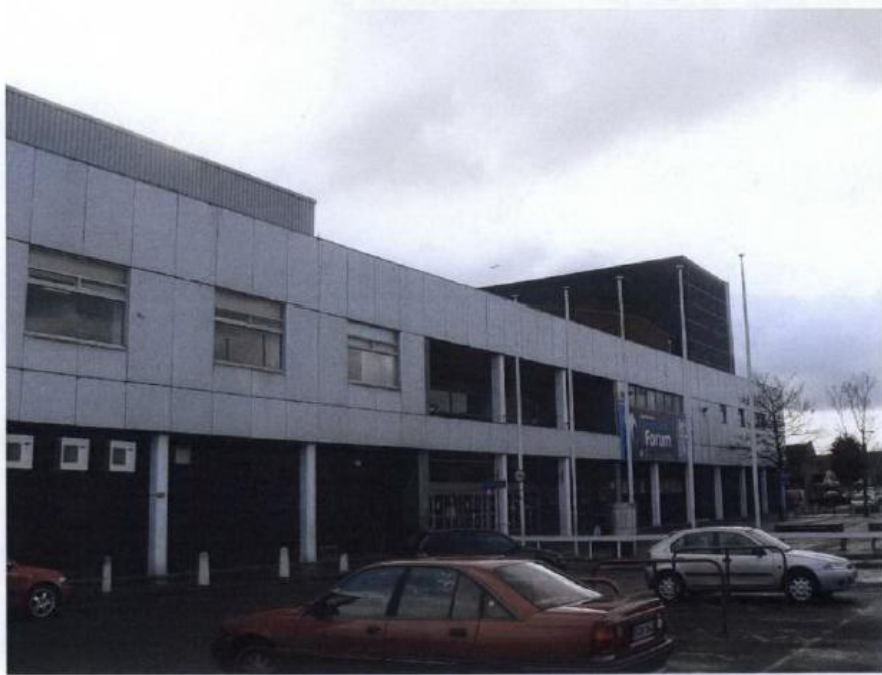
Figure 12: Old West Facade
