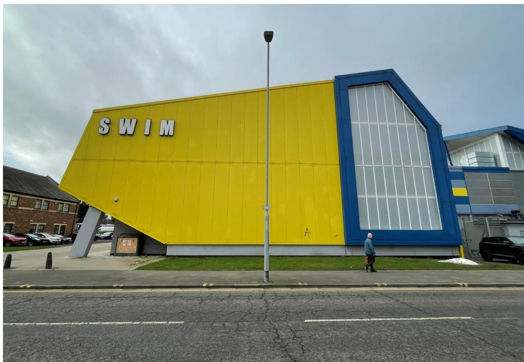
Figure 11: Current Swimming Pool Building Fabric
