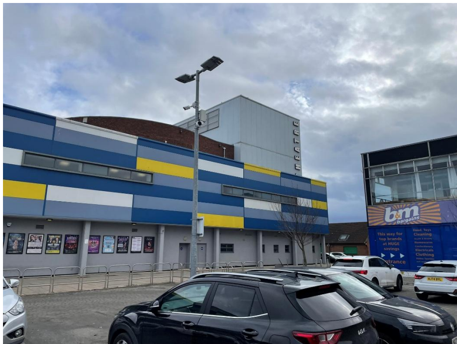
Figure 13: Existing Modern West Facade
