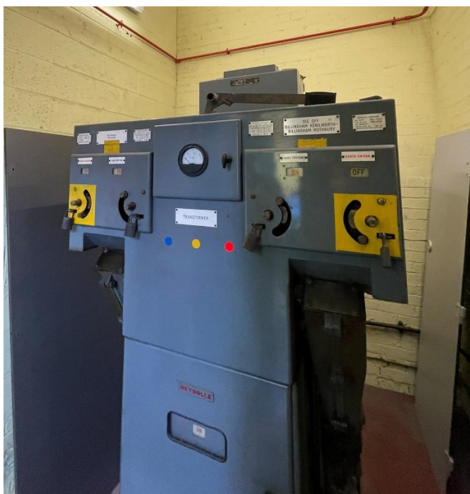
Figure 48: Main Site Transformer and Incoming Meter
