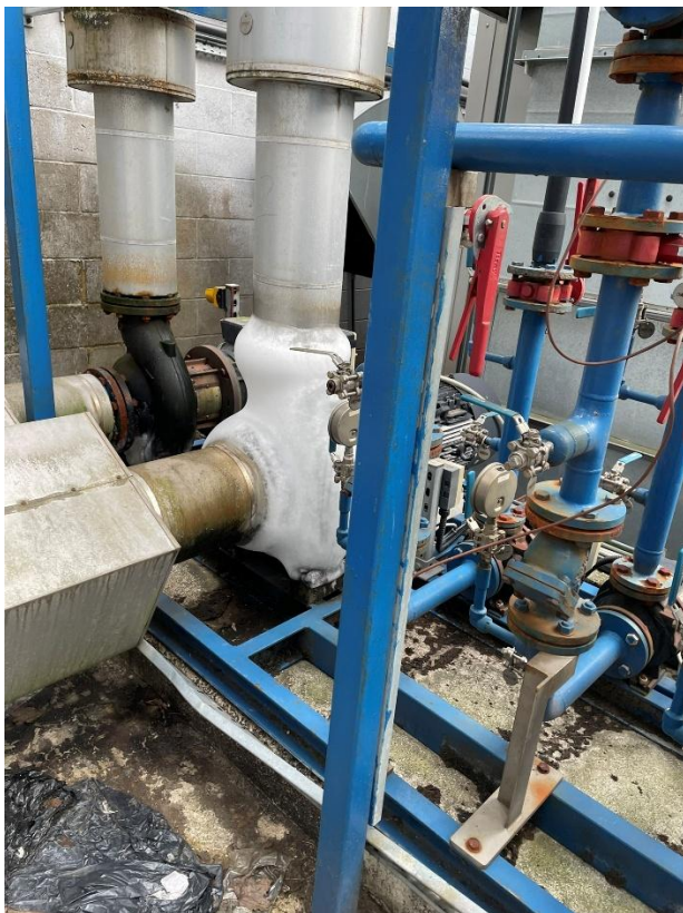
Figure 53: Frost build up on the Refrigerant Pipework
