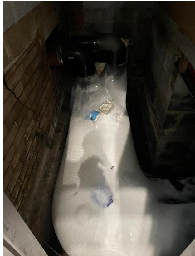
Figure 53: Frost build up on the Refrigerant Pipework
