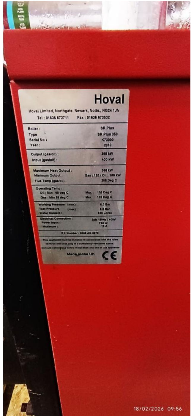
Figure 8: 3no. Hoval SR Plus 360 Oil Fired Boilers
