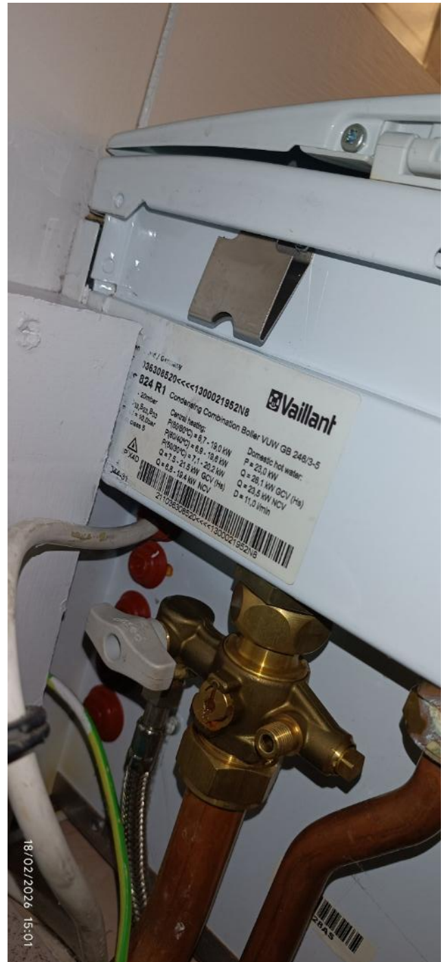
Figure 10: Anytown 2011 Extension Vaillant Gas Combi Boiler
