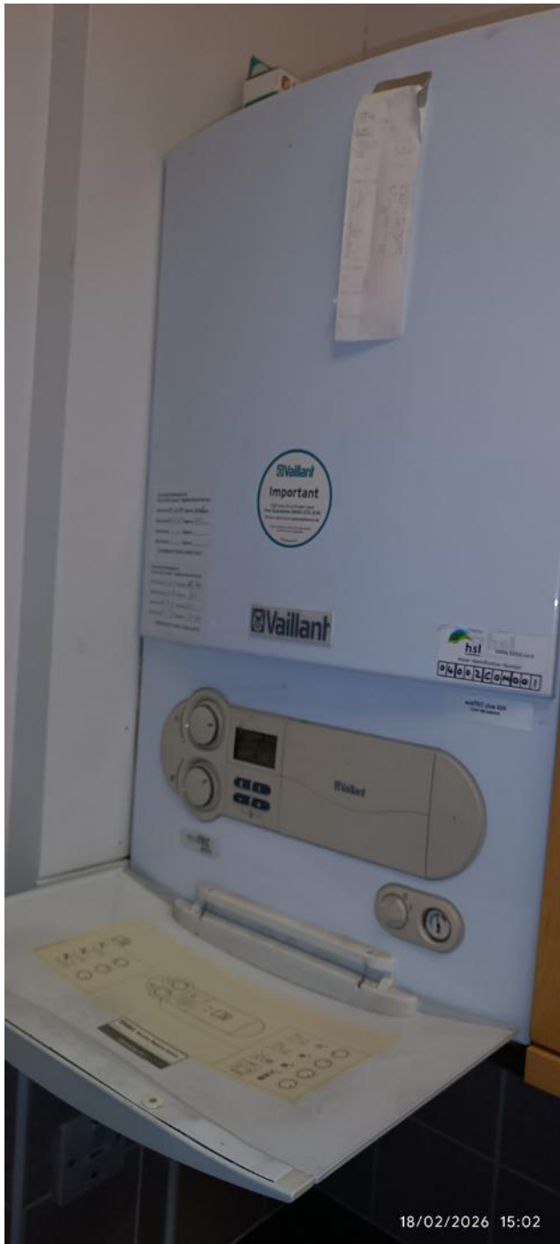
Figure 10: Anytown 2011 Extension Vaillant Gas Combi Boiler
