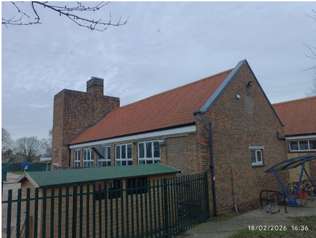
Figure 6: Newly Installed Roof Tiling
