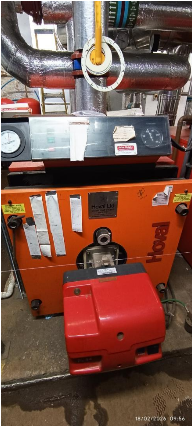
Figure 8: 3no. Hoval SR Plus 360 Oil Fired Boilers
