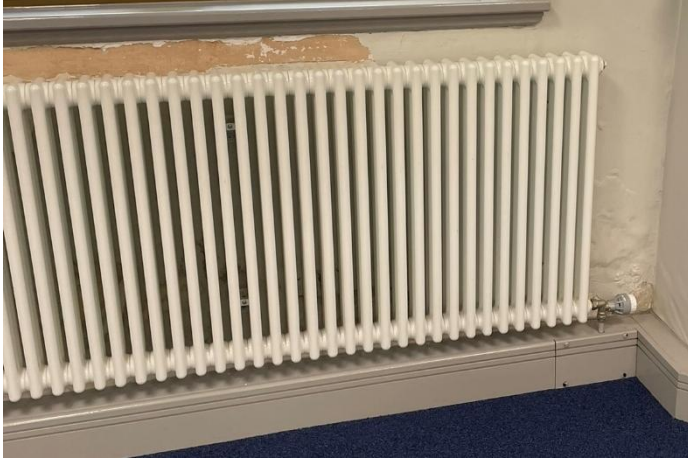
Figure 14: Different Radiator Types in the Building
