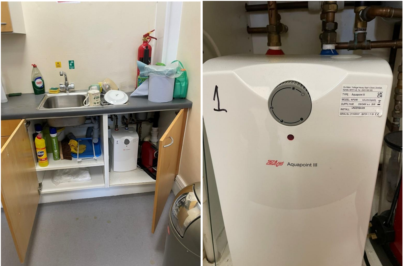
Figure 16: Point of Use Water Heater
