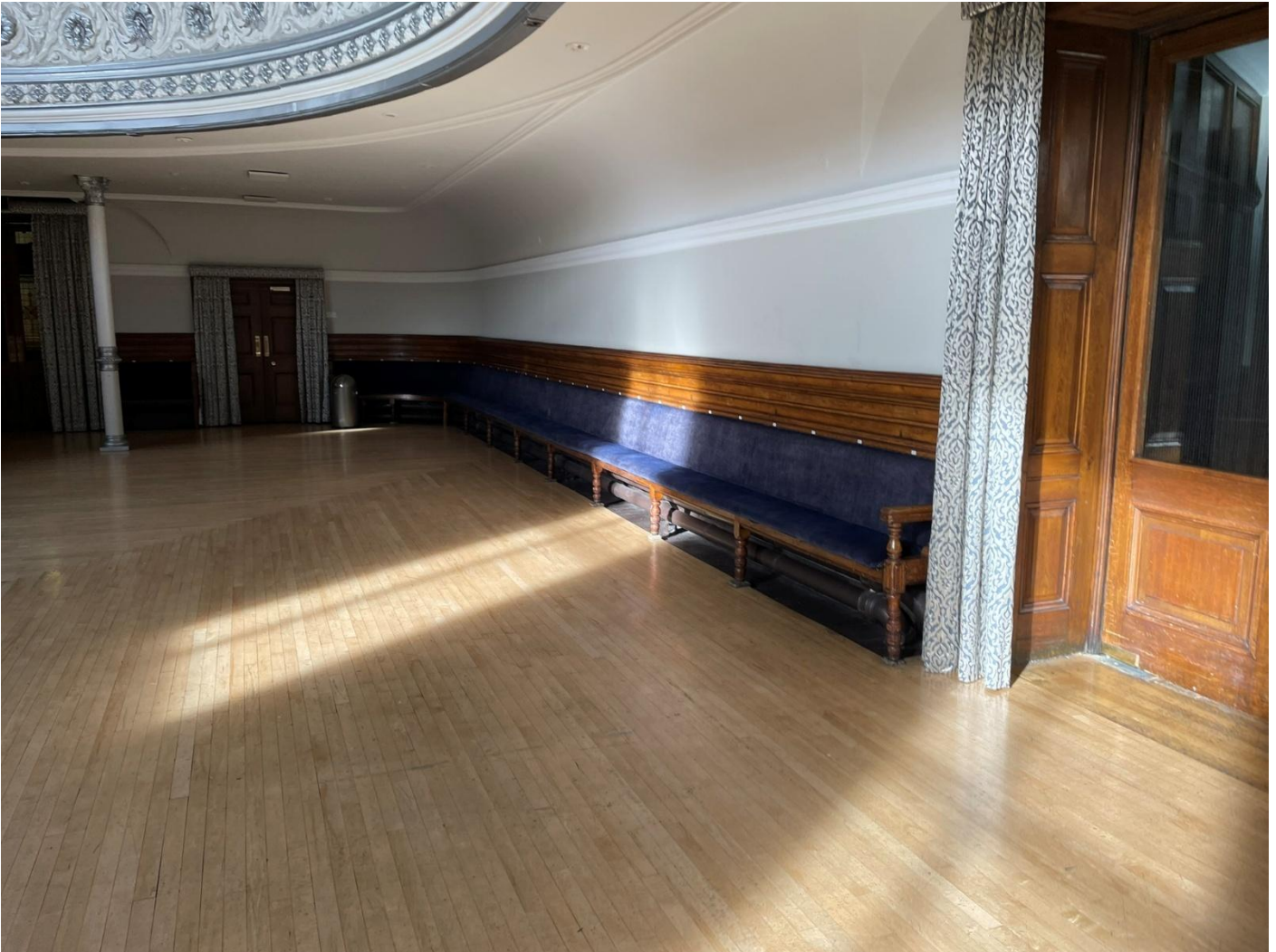
Figure 15: Heating Pipework in Victoria Hall
